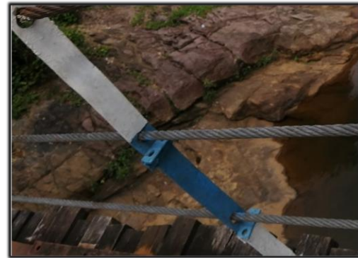
Figure 6: Cross section and image of middle and bottom wire ropes of the handrail
