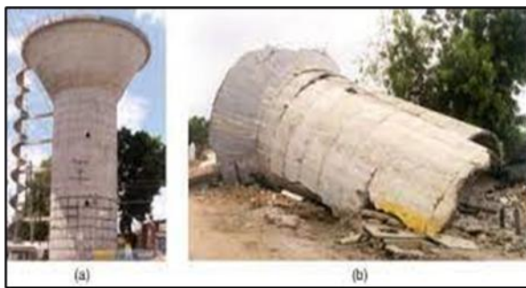
Figure 2: Water tower collapse during Bhuj earthquake in India ( Rai (2003) [4] )
