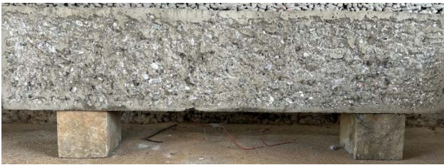
Figure 6: Roughened RC Beam Surface
