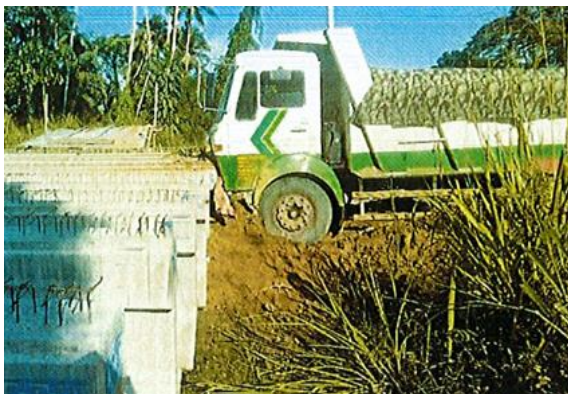
Figure 1: PSC girder stored on-site after impact by a truck.
