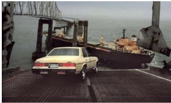
Figure 2: Sunshine Skyway Bridge collapse after vessel collision [6]
