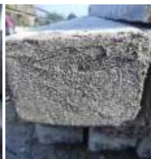
Figure 5: Top end of the electricity pole after plastering
