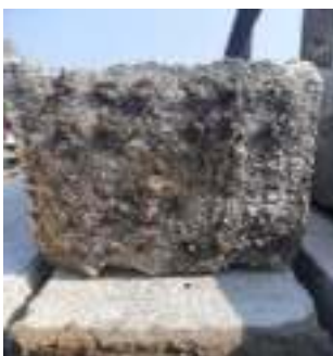
Figure 4: Top end of the electricity pole before plastering
