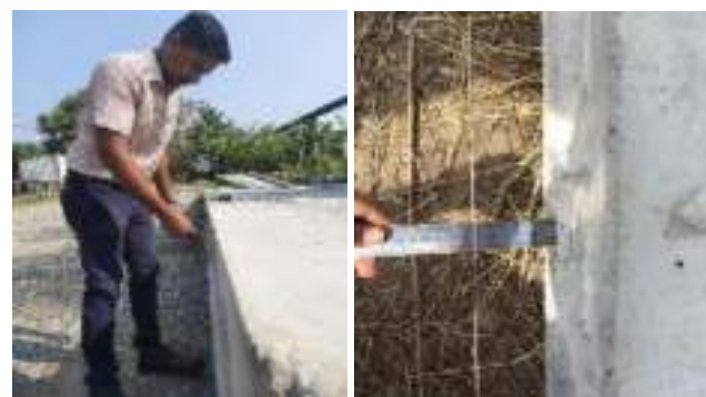
Figure 1: Getting measurements of lateral deformations in electricity poles
